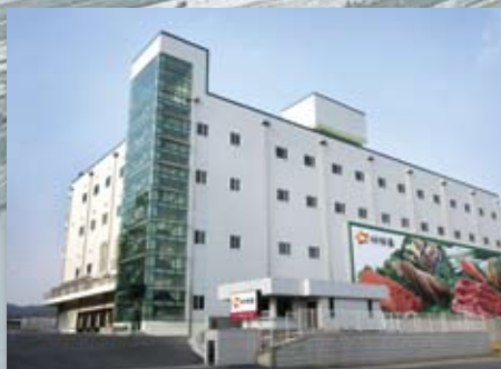
Yongin Factory 2 / Logistics Center #263 Gyeonggidong-ro, Namsa-myeon, Cheoin-gu, Yongin, Gyeonggi-do
